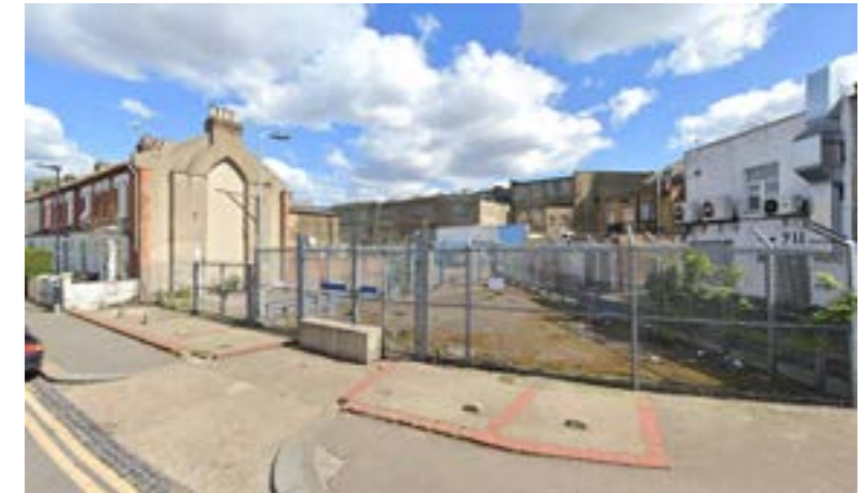
Existing view from Suffield Road
